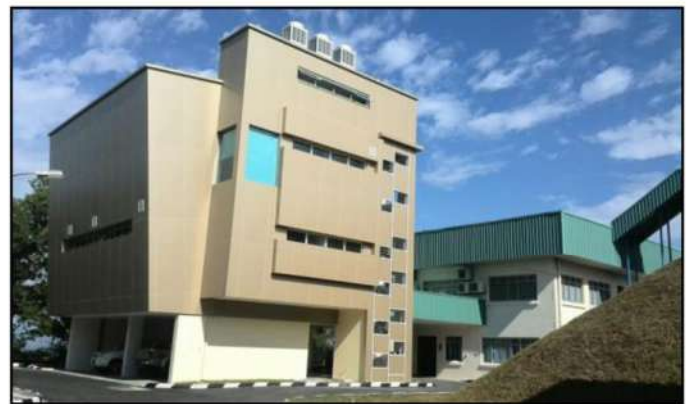
Water Treatment Plant (Mengkabau)
