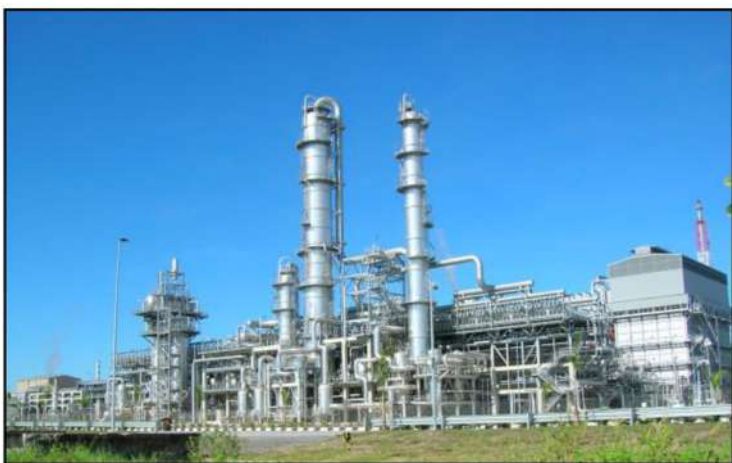
Brunei Methanol Complex (SPARK)
