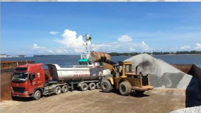
1) Aggregates arrive via barge
