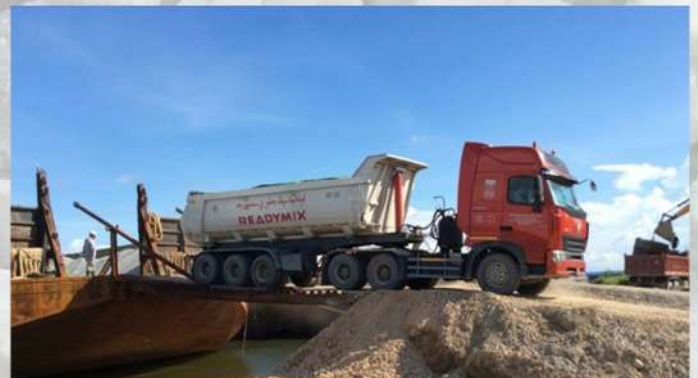
2) Transportation of aggregates to stockpile by Readymix Tipper Truck
