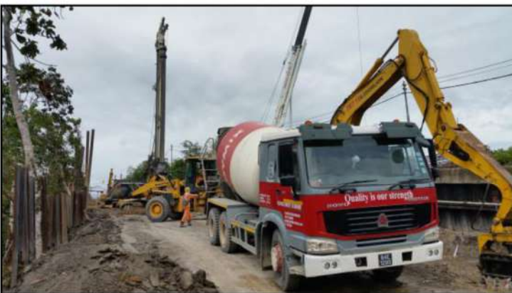
Slope retaining wall (Jln Tutong)
