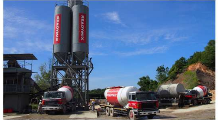
2) Transportation of cement to Readymix plants. Cement is then pumped into silos by pneumatic blower through a pipe mounted on the side of silos
